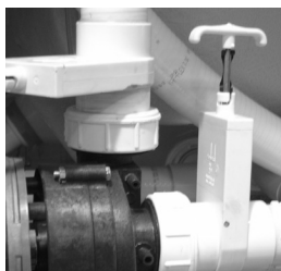
Slice Valve and Pump Union
